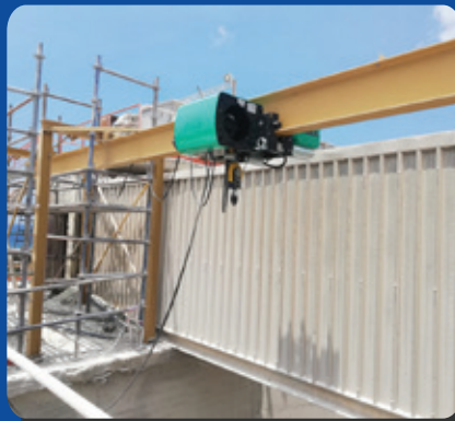
SLCB Crane - Chekka
