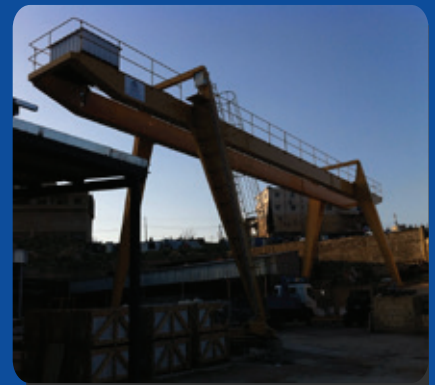
Rafli Diab & Co - Gantry Crane - Kaferkahel
