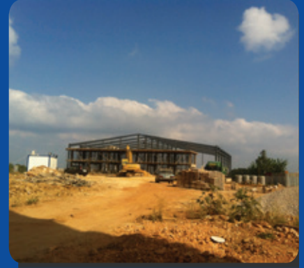
Makhazen Warehouse - Chouwaifet
