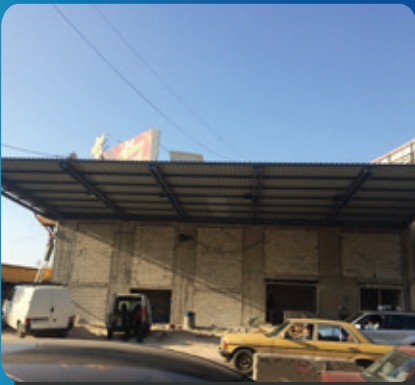
Medco Station - Bahsas
