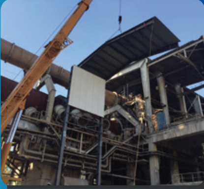
Holcim Kiln Tent - Chekka
